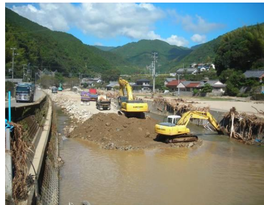
Figure 18: Emergency removal of earth from waterways
