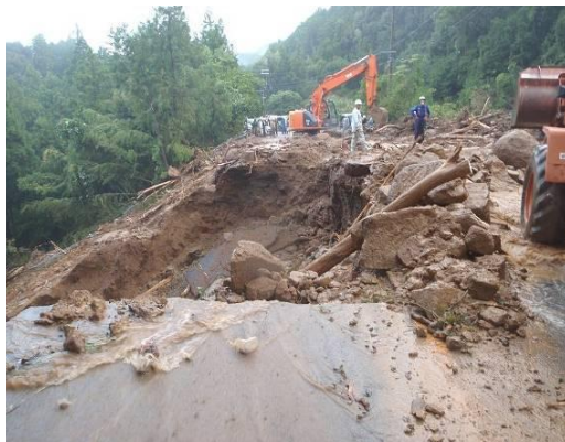
Figure 17: Emergency works on a collapsed road
