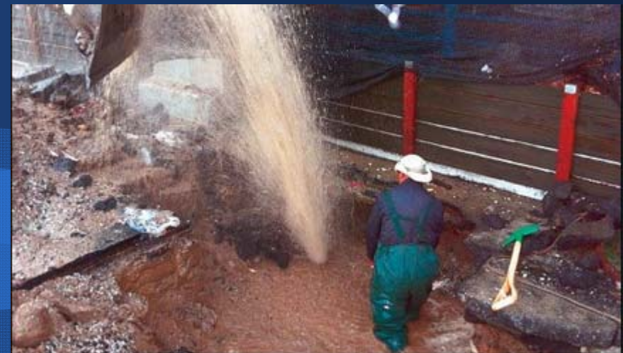
<Bursts of Water supply system in Seoul>
