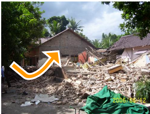
Figure 3: Two examples of the application of BARRATAGA concept by trained mandors. The two houses have stood completely with very light cracks surrounded by heavy damaged and collapsed regular houses due to the 2006 Yogyakarta-Central Java earthquake (Sarwidi et. al., 2007)
