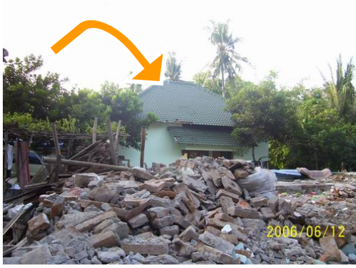
Figure 3: Two examples of the application of BARRATAGA concept by trained mandors. The two houses have stood completely with very light cracks surrounded by heavy damaged and collapsed regular houses due to the 2006 Yogyakarta-Central Java earthquake (Sarwidi et. al., 2007)
